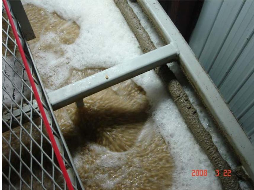
**Figure 2. Top of the MBBR tank indicating foaming problem.
